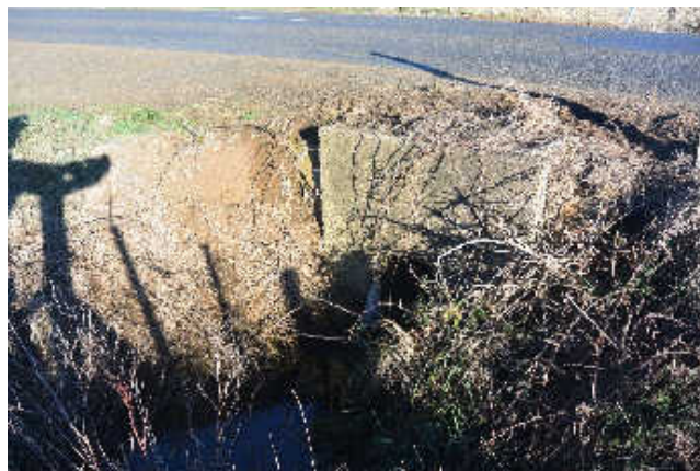
Fig. 2 Vegetation killed on steep embankments around culvert intakes leads to erosion of soil and gravel – pollution of watercourses by suspended particles – siltation of our estuaries.
