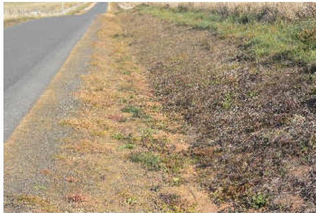
Fig. 1 Road verge and table drain sprayed twice to clear vegetation. Storm water runoff can flush pollutants from road surface directly via drains into our creeks without first filtering through a grassy filter strip.
