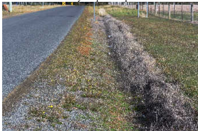
Fig. 2 Vegetation killed on steep embankments around culvert intakes leads to erosion of soil and gravel – pollution of watercourses by suspended particles – siltation of our estuaries.
